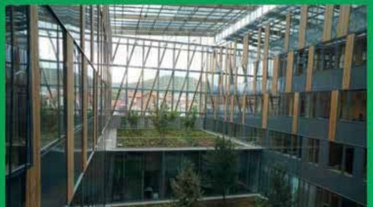
HOTEL DE REGION AUVERGNE - CLERMONT FERRAND Architecte: Bruno Mader
